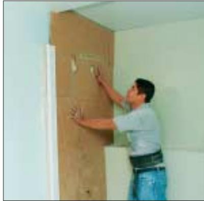
The first step in a typical installation (a shower surround is installed here) is to make cardboard templates of the areas so that the panels can be cut to rough size at the factory.
