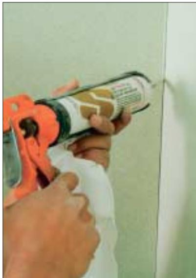
After all of the panels are installed, color-matched caulk is applied at all joints. The result is a watertight installation that requires very little maintenance.
