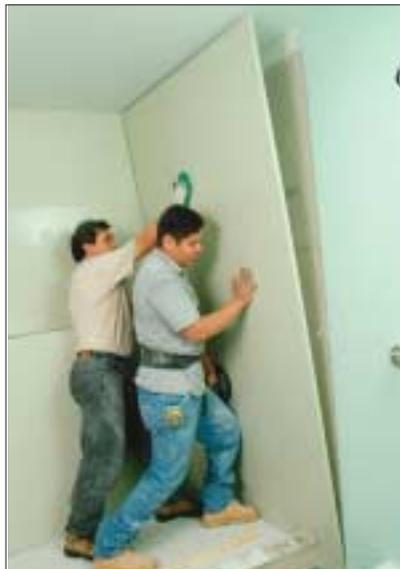
A special adhesive is applied to the backs of the panels; then they're pressed into place and braced in position while the adhesive cures.
