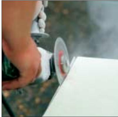
Installers make the final cuts on site to ensure a tight fit. Diamond-coated blades are necessary to cut through the hard quartz.
